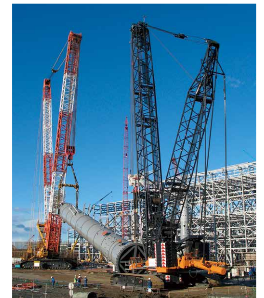
Erecting a tower on Sakhalin
