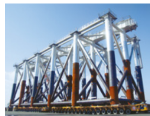
Transport of bridge piers at Tokyo International Airport
