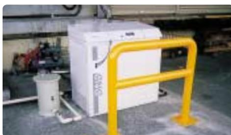
Small-scale CNG filling pump \*2
