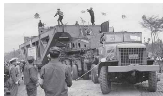
300-ton trailer on its way to the West Tokyo Power Transformer Station
