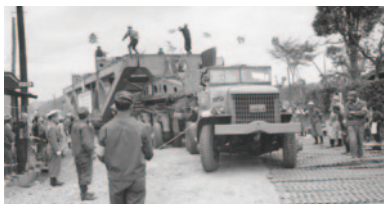
300-ton trailer on its way to the West Tokyo Power Transformer Station
