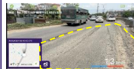
Center-lane level changes and uneven pavement
